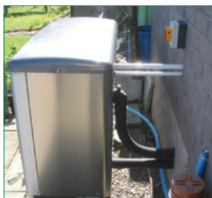
Air Source Heating Unit
