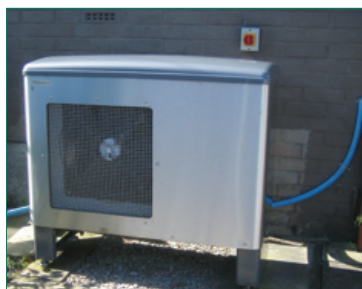
Air Source Heating Unit
