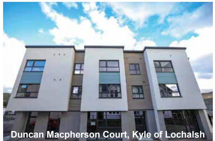
Photograph courtesy of Compass Building & Construction
